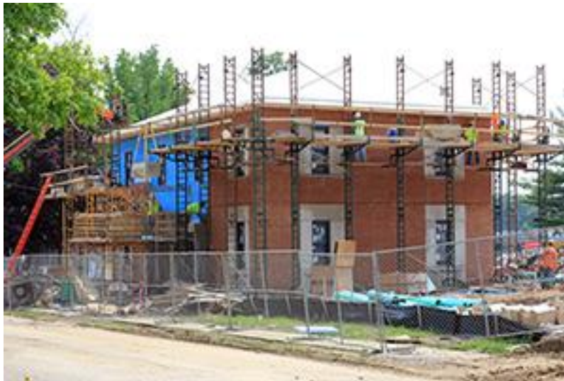
Housing Under Construction!
